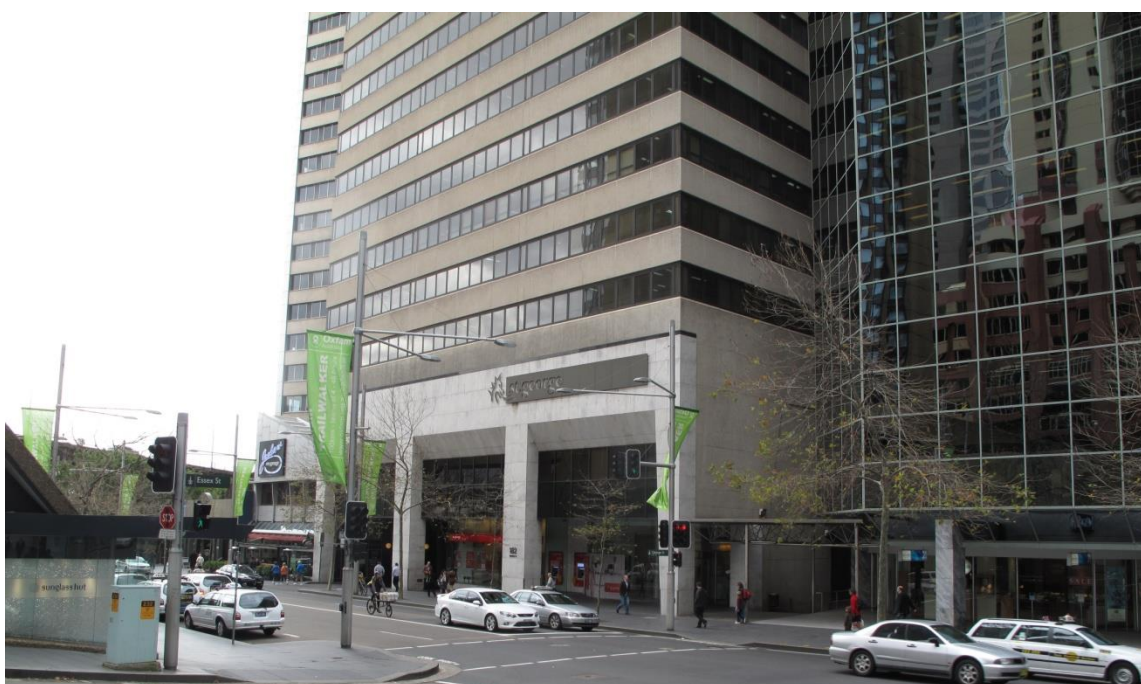
Figure 2.1: 182 George Street, centre left, looking northwest. C&L 2013.
